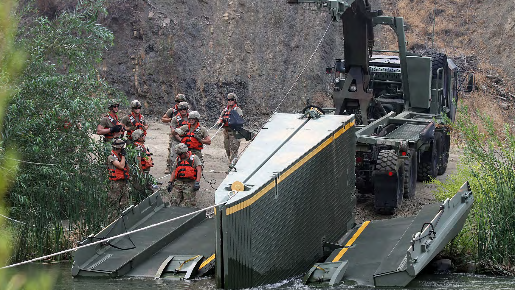
Members of the 132nd Multirole Bridge Company, 579th Engineer Battalion, 49th Military Police Brigade, unload a floating platform, at Cache Creek Canyon Low Water Bridge, Capay Valley, California.
